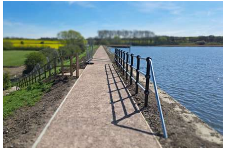
The new levelled and resurfaced crest footpath Kate Andrew
