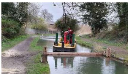
The closure at Little Tring with the stop planks in place
