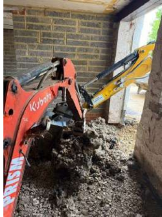
Excavation of internal floors
