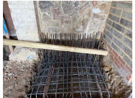
Steel reinforcement inside
