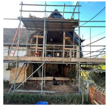
Nov. 2023 - Old, rotten timbers removed, retaining as much original fabric as possible. Replacement green oak beams starting to be installed
