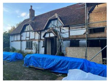
Nov 2023 - Completed roof works with new lead flashing
